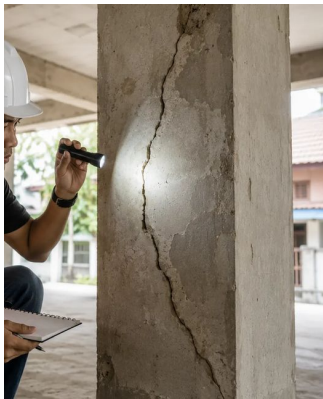
Photo 1 — O-1, diagonal crack above window W-2, north elevation, ground floor. Comparator card in frame. Illustrative photograph.
